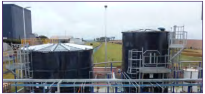
2: Tapered Beam Roof – Brazil
